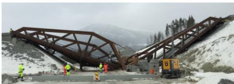
Figure 3.50 Perkolo bridge hours after the collapse (Photo: R. Abrahamsen)
